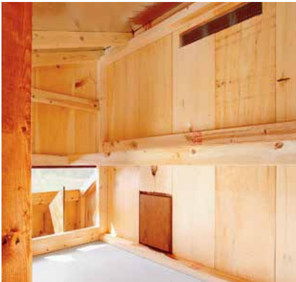
Interior view of L35 (page 47)
