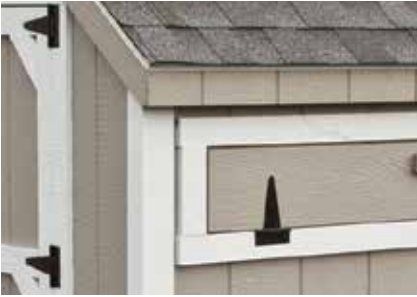
Shown Here: Light Gray Siding with White Trim
